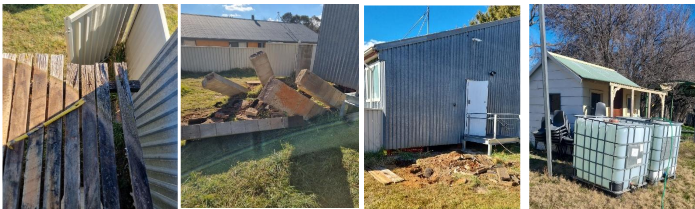
Above: 1. Dodgy wooden platform under old tank. 2. Concrete pillars for platform support. 3. The almost-cleared site. 4. Some water for the new tank, supplied by Allan.
