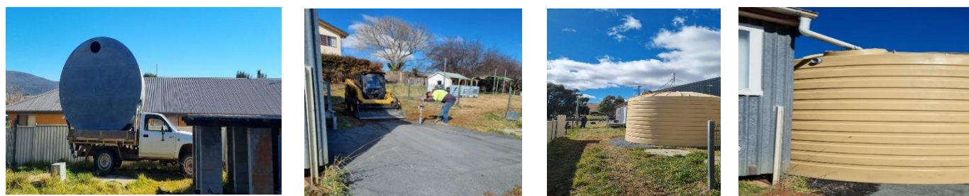
Above: 1. Goodbye to the old tank. 2. Base for the new tank being prepared. 3. Helpers had to remove the side fence and gate for the new tank's entry, then reconstruct them, including concreting the posts. 4. The glorious new tank waiting for rain.
