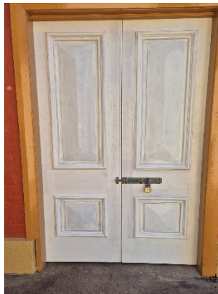
Above: The sanded and resurfaced kitchen floor, the reconstructed doors of the storage room (awaiting paint), and the rehabilitated original handle on the kitchen door. This is all impeccable work by heritage craftsman Myles Gostelow of Tharwa.
