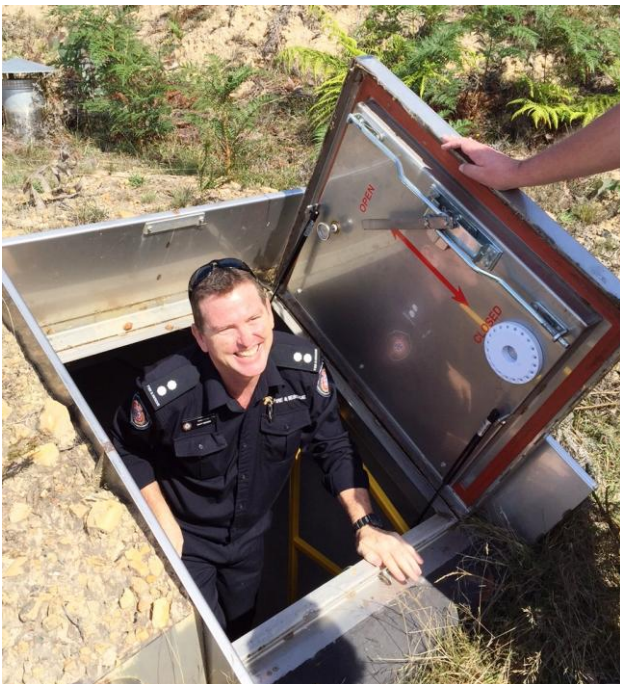
Bunker to protect fire spotters, at the base of the Millgrove (Vic.) fire tower: (photo: Sandra)
